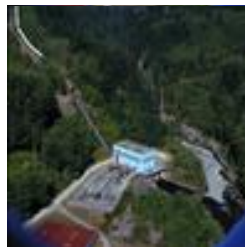
Jordan river power house
