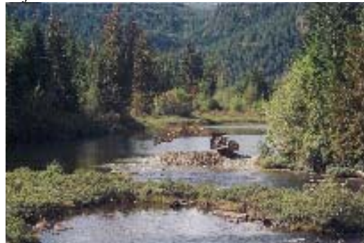
Photo 12. Upstream view of platform A construction, Dickson Lake outlet.
