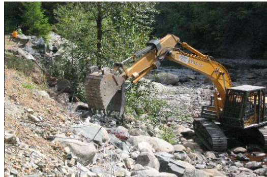
Photo 24. Armouring disturbed stream bank, South Nanaimo River.
