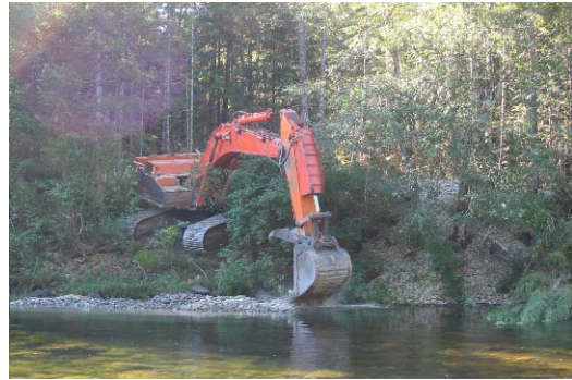
Photo 16. Excavator placing material into outlet channel, Nanaimo River.
