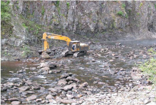
Photo 19. Excavator building route for front-end loader, South Nanaimo River
