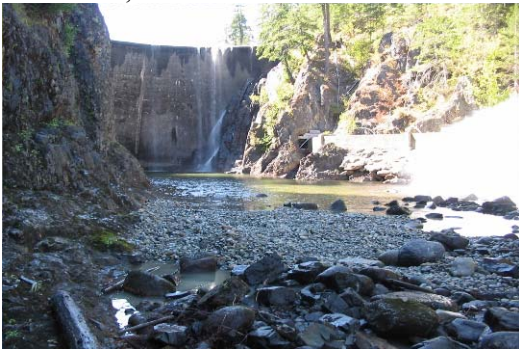
Photo 23. Upstream view of Site #3, South Nanaimo River.
