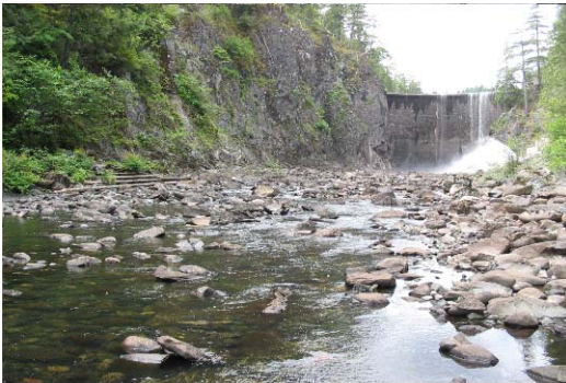
Photo 3. South Fork Dam, South Nanaimo River.
