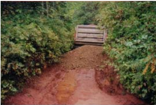
Photo 11. Road grade improvements at campsite near Dickson Lake outlet (left bank).
