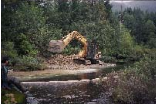
Photo 13. Upstream view of platform B construction, Dickson Lake outlet.
