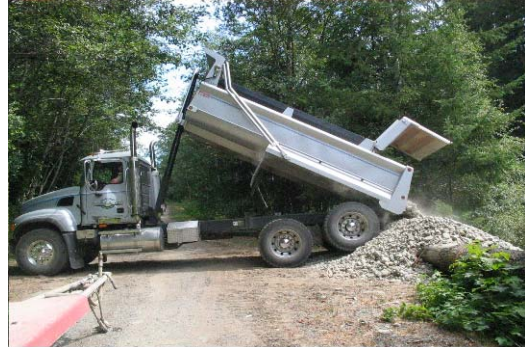
Photo 10. Gravel delivery down steep bank adjacent to South Nanaimo River.
