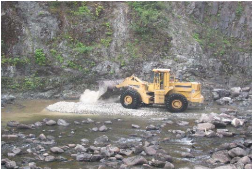
Photo 21. Front-end loader moving material into Site #2, South Nanaimo River.
