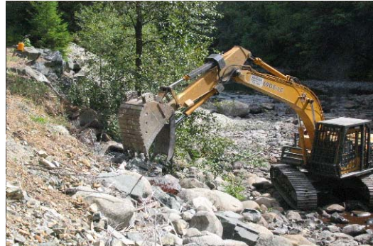
Photo 24. Armouring disturbed stream bank, South Nanaimo River.
