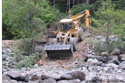
Photo 20. Access route into South Nanaimo River channel.
