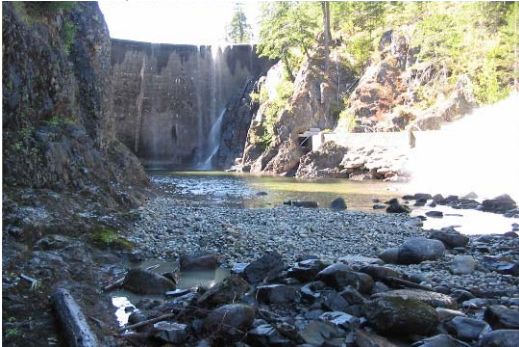
Photo 23. Upstream view of Site #3, South Nanaimo River.
