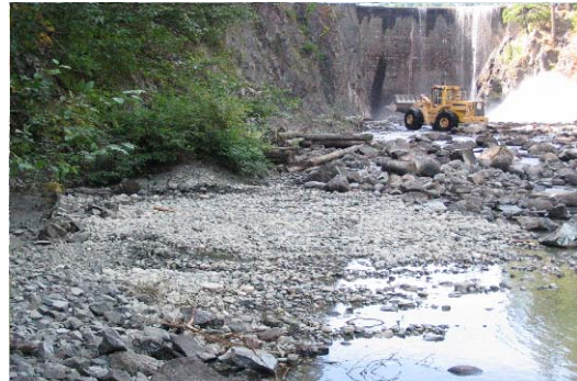
Photo 22. Upstream view of Site #2, South Nanaimo River.
