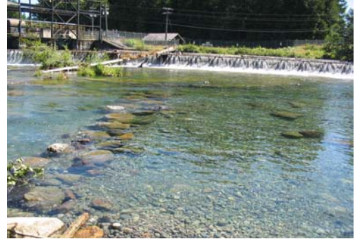
2. Completed spawning platform at Site 1 (Diversion Dam).
