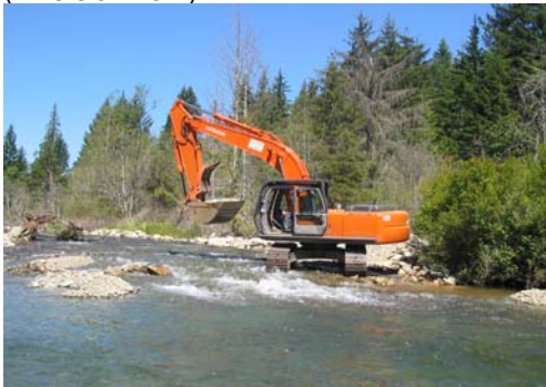
3. Gravel placement by excavator at Site 2 (Bull Island Side-channel).
