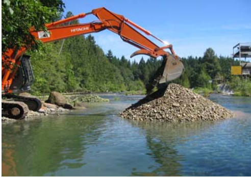
1. Gravel placement by excavator at Site 1 (Diversion Dam).
