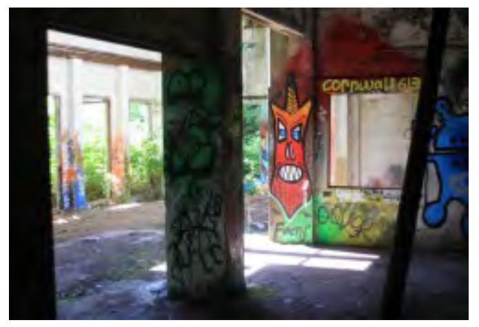
Last century the Jordan River once had a power station that generated electricity for part of Victoria
