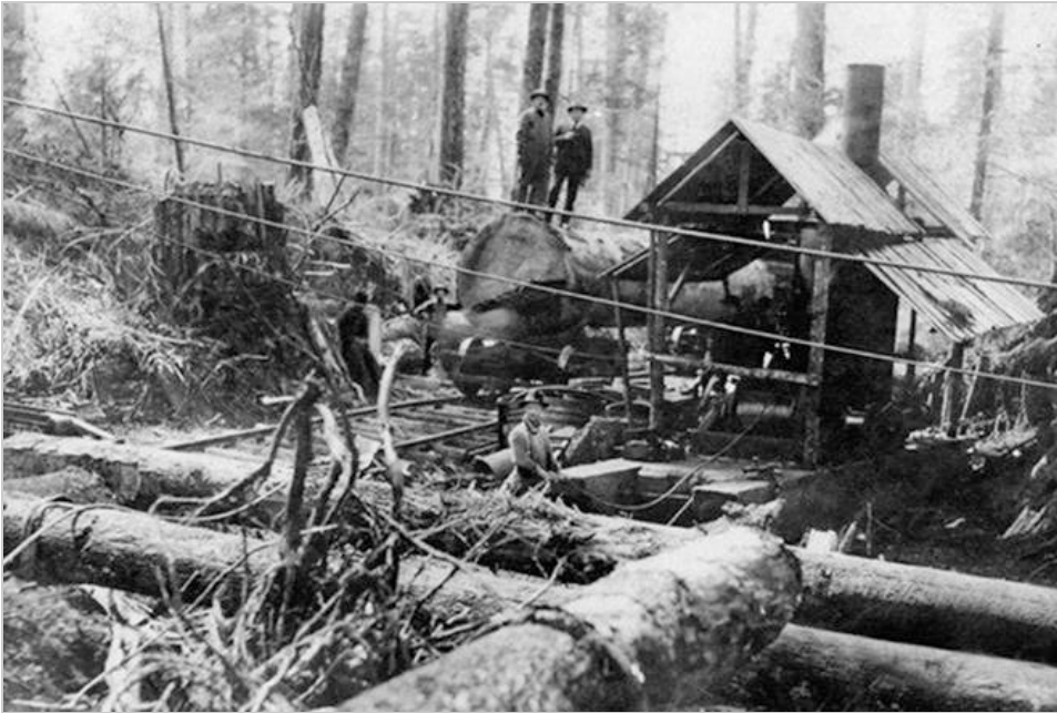
The photo shows a steam donkey engine yarder and cables alongside the logging railway in Jordan River. (Sooke Region Museum)
