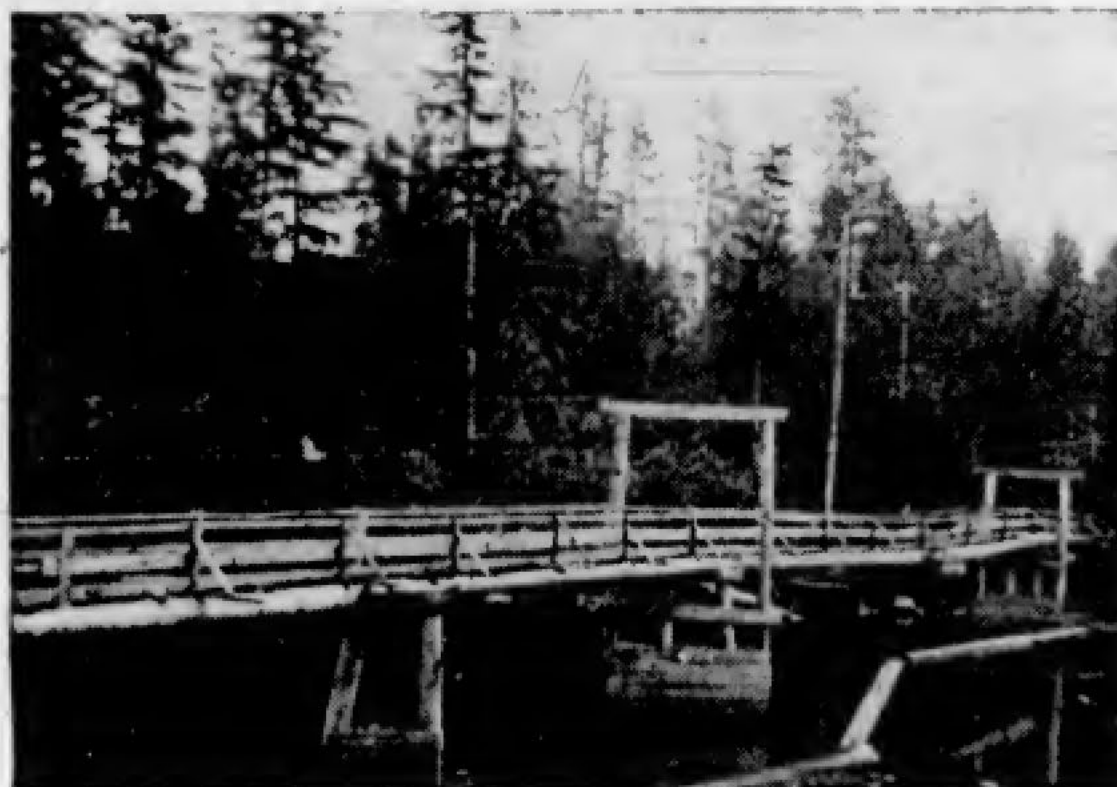
The Old Bridge at Jordan River Mouth.
