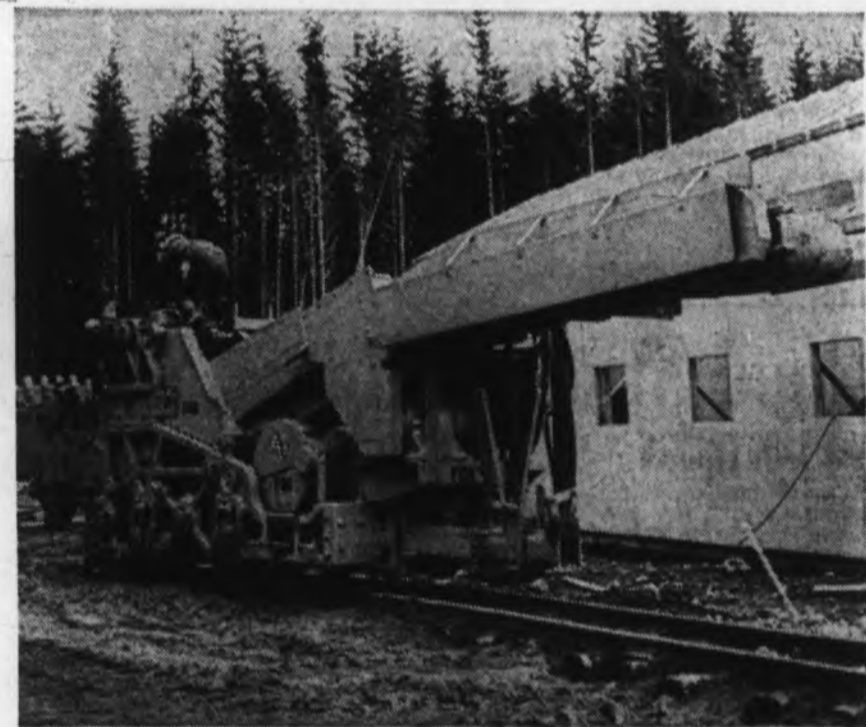
Mucker moves in after blast, clears debris into rail cars
