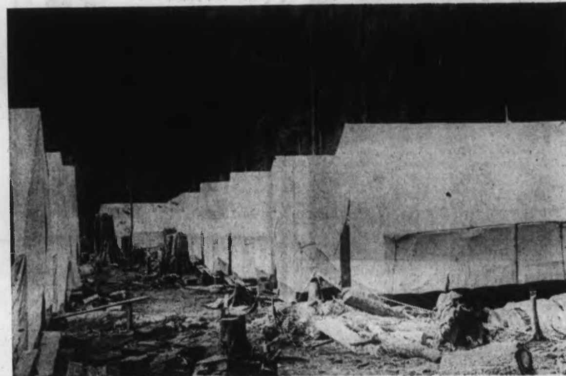
An early day construction camp at Jordan River project
