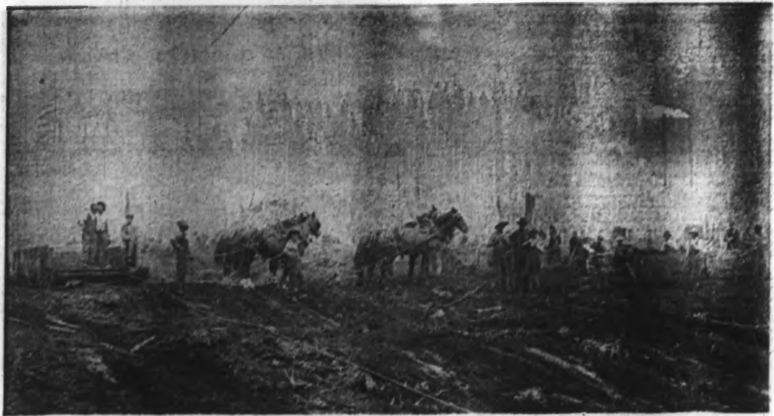
JORDAN RIVER MAY SOON COME ALIVE AGAIN as workers seek reconstruct hydro plant, pictured here under construction in early 1900s.
