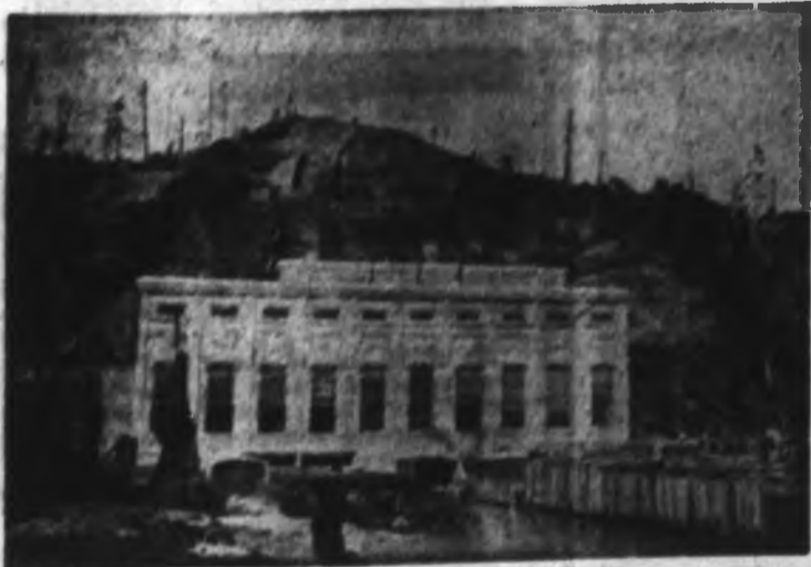
JORDAN RIVER POWER HOUSE AND TAILRACE.
