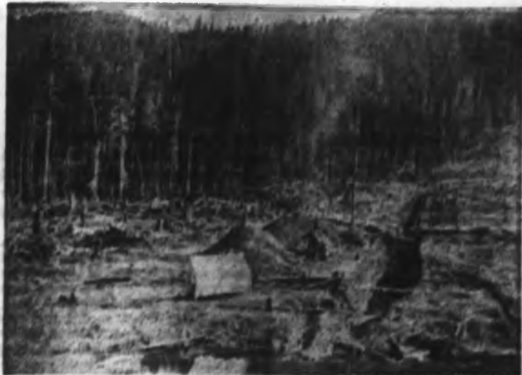
START OF BEAR CREEK DAM.
