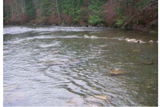
2. Completed spawning platform at Site 1 (Barber's Pool).
