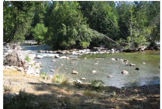
4. Completed spawning platform at Site 2 (upstream Bull Island Side-channel intake).
