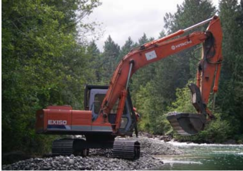
1. Gravel placement by excavator at Site 1 (Barber's Pool).
