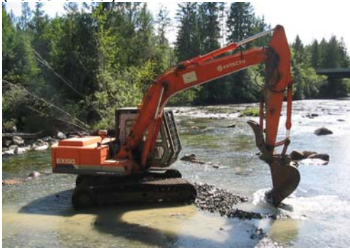
3. Gravel placement by excavator at Site 2 (upstream Bull Island Side-channel intake).
