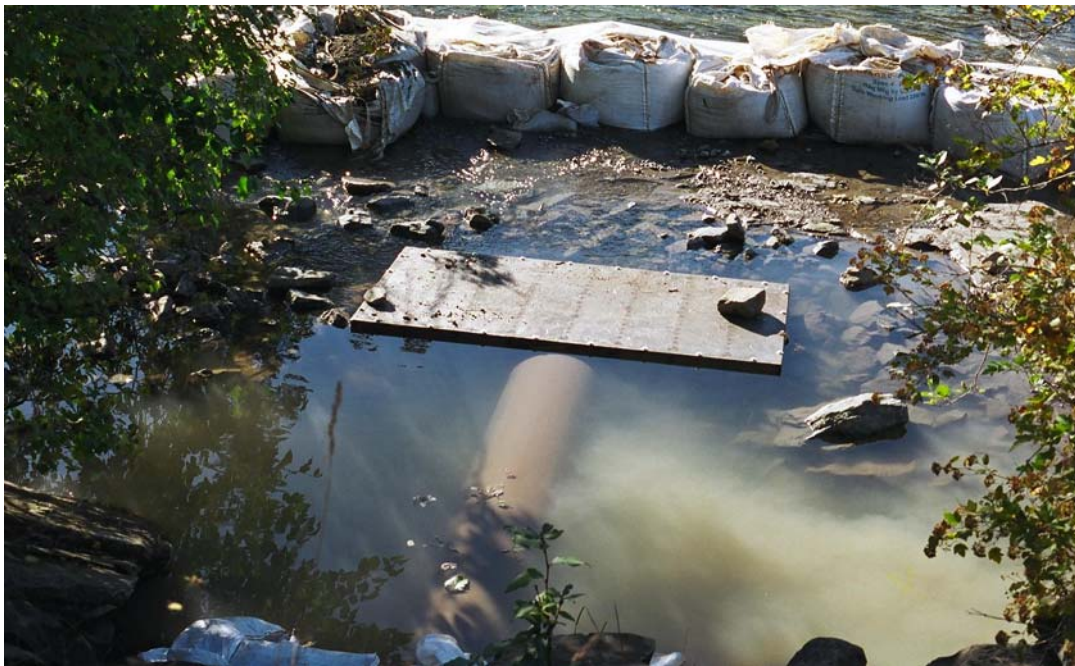
Photo 2. New screened box intake isolated from river during installation in 2003.
