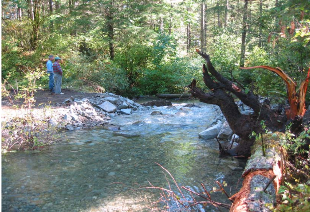
Photo 3. Looking downstream at new rock weir and spawning platform located approximately 150 m downstream of intake.
