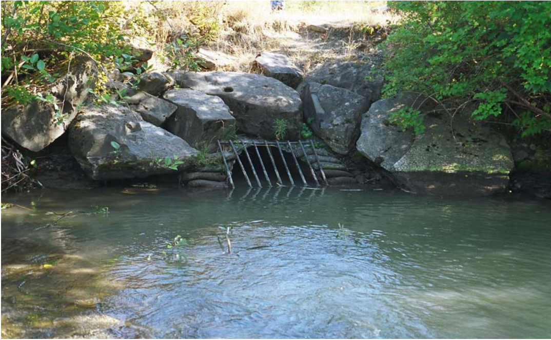
Photo 1. View of the original intake into the Powerline side-channel taken from the mainstem river.
