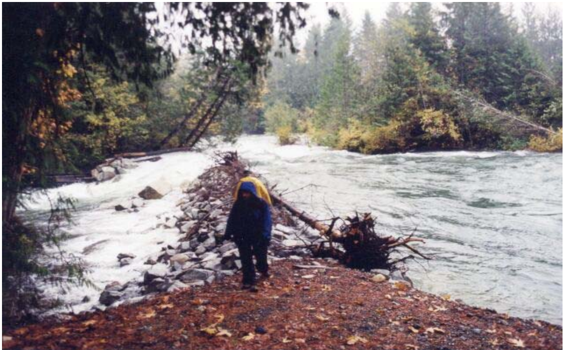
Photo 4. Deflector groyne performing at high flows in the Puntledge River, October 2003.
