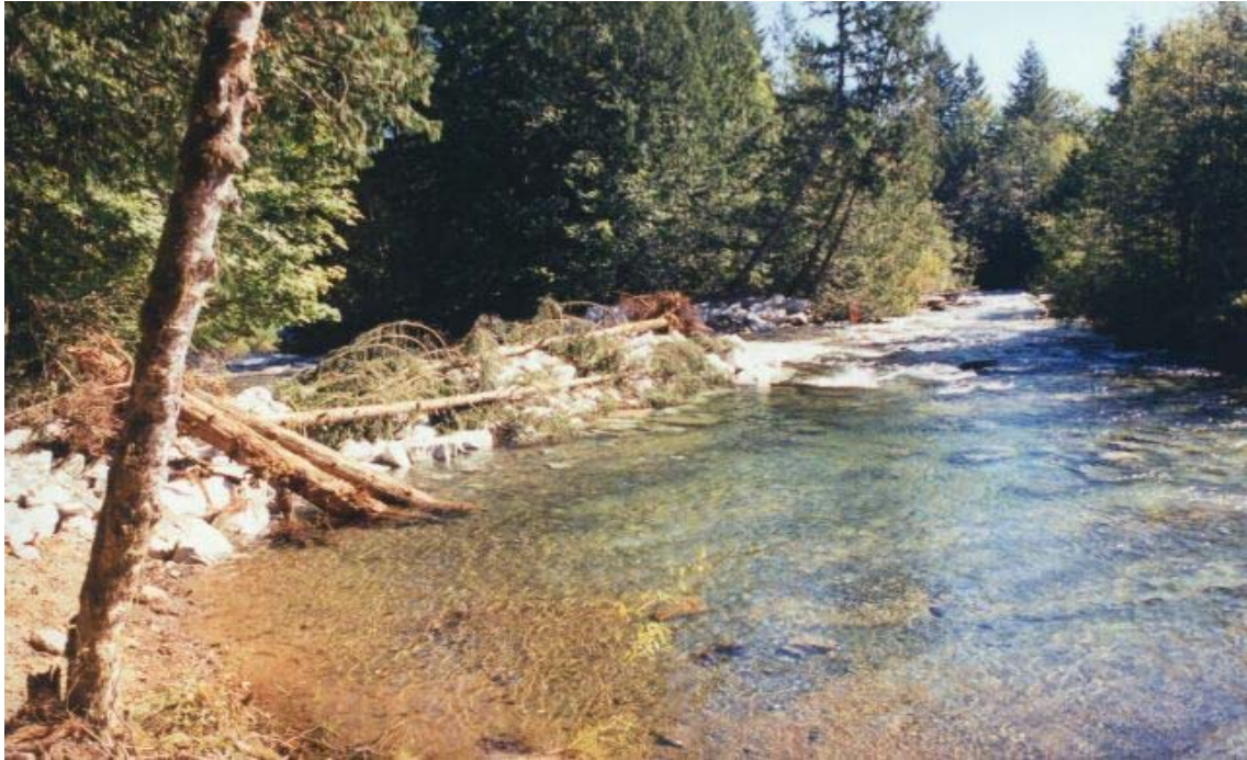
Photo 3. Deflector groyne at the entrance to the Bull Island side-channel (from left bank).
